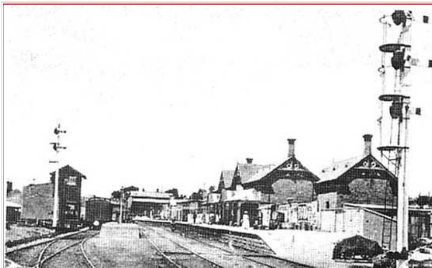
Murray Bridge Station 1910 The Signal Cabin is on the left
